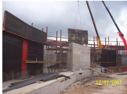
Fig.4 The 1m thick concrete slab
