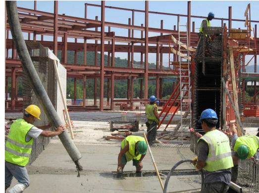
Fig.3 Concrete being poured in a slab sector
