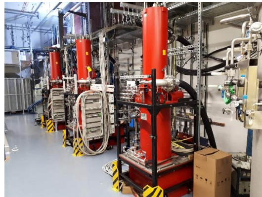
Power supply room (left) and klystron gallery (middle). In the right picture you see the klystron and the AFT circulator (left bottom) and the 300 kW load (left top)
